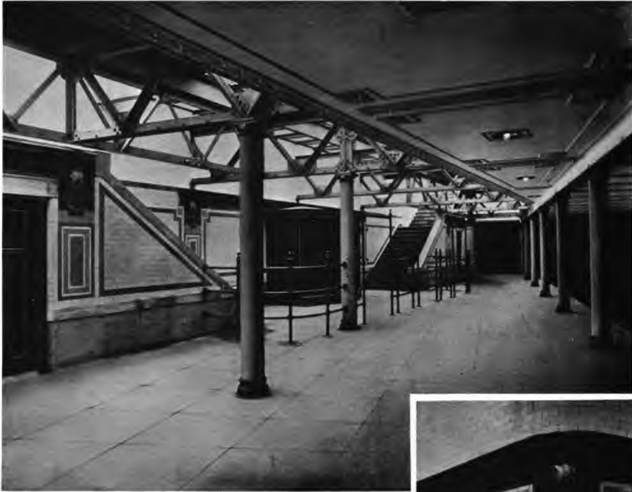
WEST SIDE OF COLUMBUS CIRCLE STATION (60TH STREET) — ILLUMINATED BY DAYLIGHT COMING THROUGH VAULT LIGHTS
